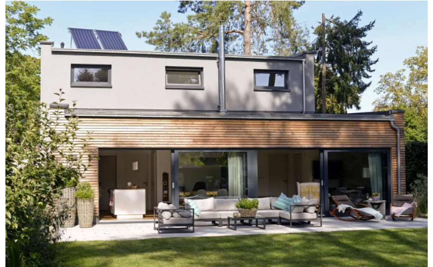
SOLAR HOME SYSTEM
