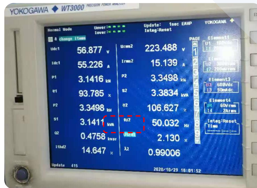
Utility Power factor 0.99
